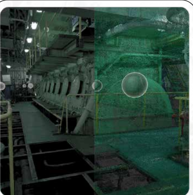
3D Scanning surveys of Ship's Engine Room and internal structures, using LIDAR equipment, 3D modelling based on Point Cloud data.
